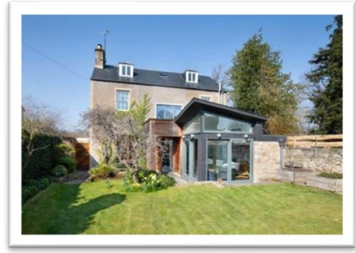
Figure 19 Rear of Lyme House
