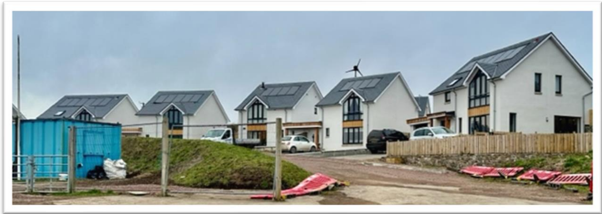
Figure 27 1 3/4 Storey Gable fronted properties near Peebles
