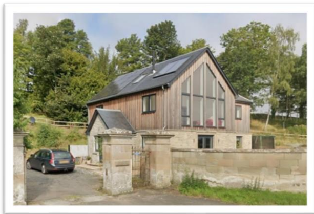
Figure 26 Two Storey Glass gable property Coldstream Road
